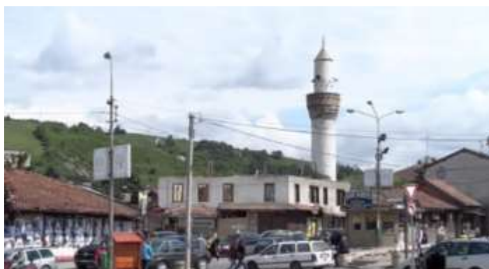
Fig. 2. Arab mosque in the first phase of demolition
