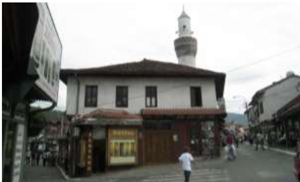
Fig. 1. Arab mosque in its original state
