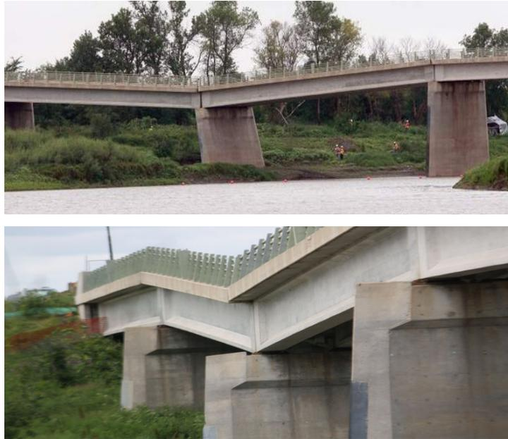
**Fig. 1.10** Failure of the St. Adolph Bridge, Winnipeg, Canada, 2009
