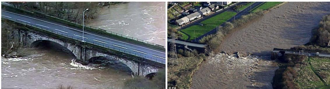
**Fig. 1.7** Northside Bridge prior and after the failure, Workington, UK, 2009
