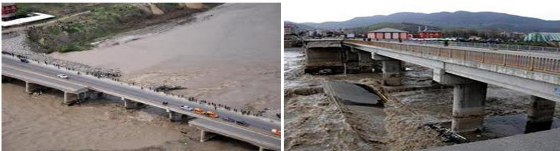
**Fig. 1.11** Failure of the bridge on the river Filyos, northern Turkey, 2012
