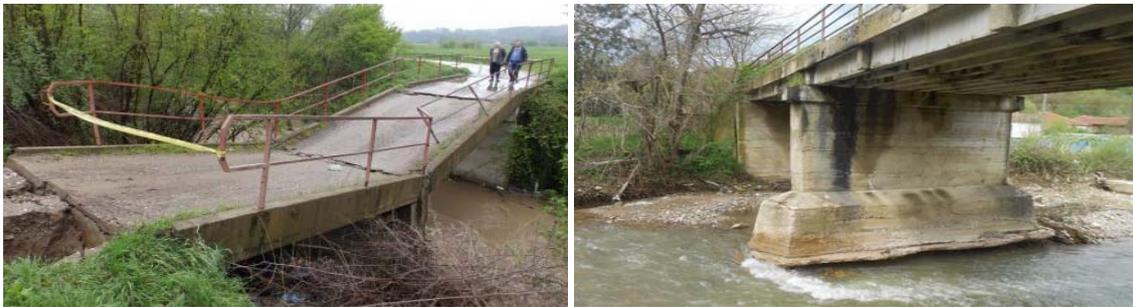
**Fig. 1.16** Bridge failure near Kraljevo (left) and scour-critical bridge near Vranje (right), Serbia, 2014
