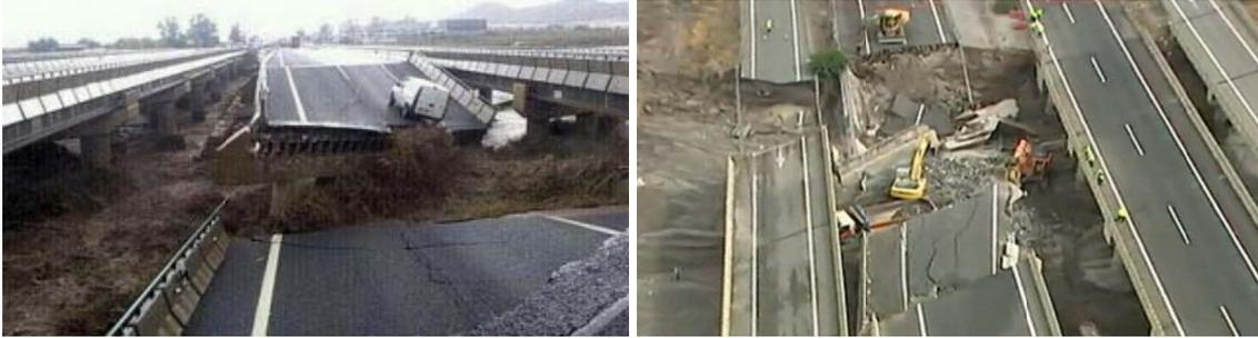
**Fig. 1.12** Failure of the bridge across Rambla de Béjar, Spain, 2012
