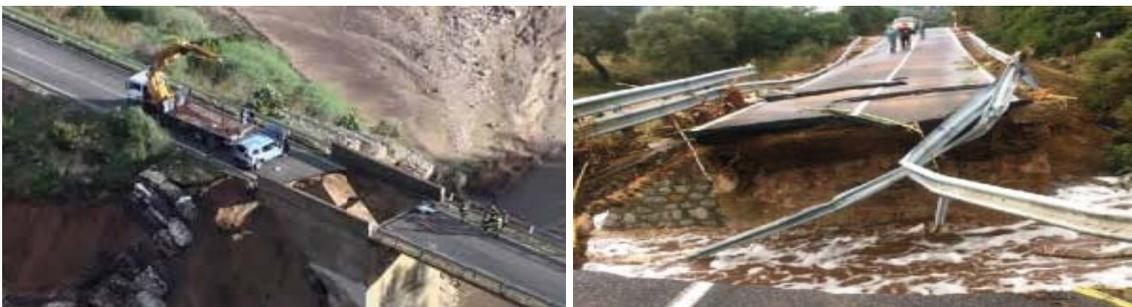
**Fig. 1.14** Bridge failures near Dorgali (left) and Olbia (right), Sardinia, 2013
