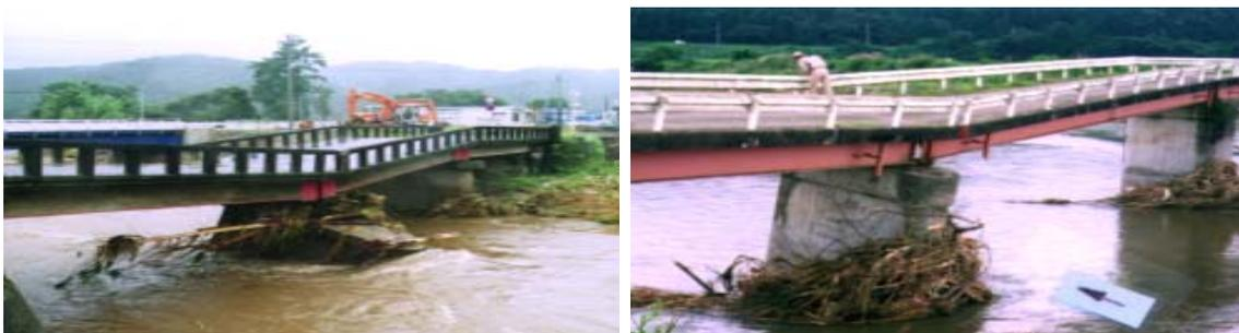
**Fig. 1.1** Bridge failures in the Kanto region, Japan, 1998, [Fukui and Nishitani, 2002]
