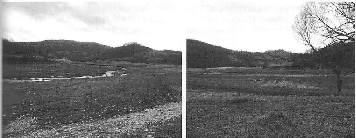
Figure 5. The most upstream part of the reservoir with sediment deposits revealed when the water level is lowered, either as an activity in flood management strategy, or due to hydropower utilization. This part of reservoir could serve as a habitat for water plants which can have an active role in intercepting incoming pollution and nutrients.
