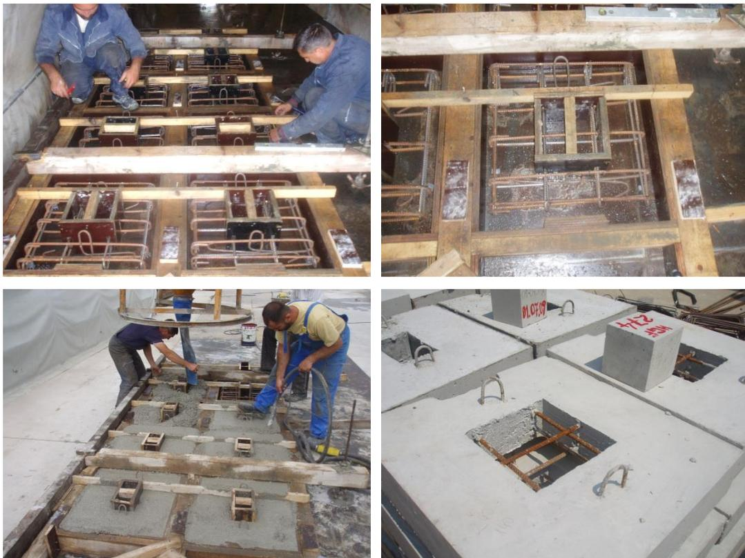
**Fig. 4.3** Prefabrication of concrete slabs in GEMAX concrete plant.
