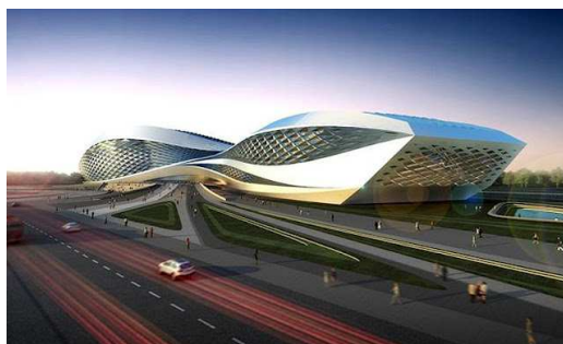
Sl. 99 The Chengdu Contemporary Art Centre (CCAC)- Zaha Hadid Architects
