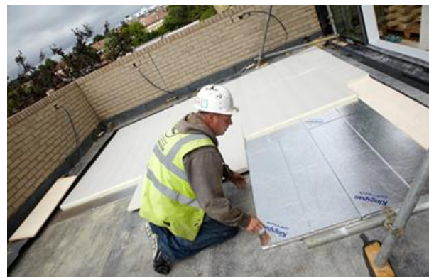
Figure 8. Example of using OPTIM-R for floor insulation [11]
