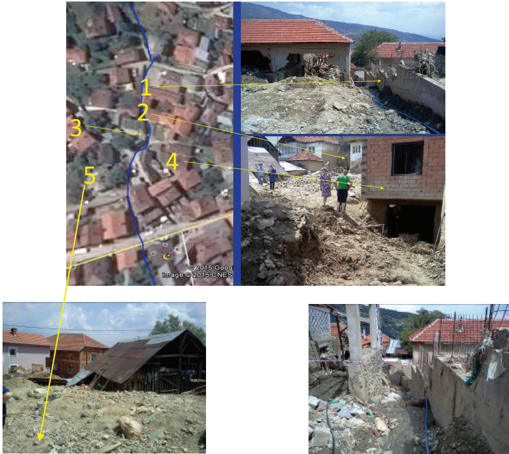
Figure 12. Location of structures along the torrent
