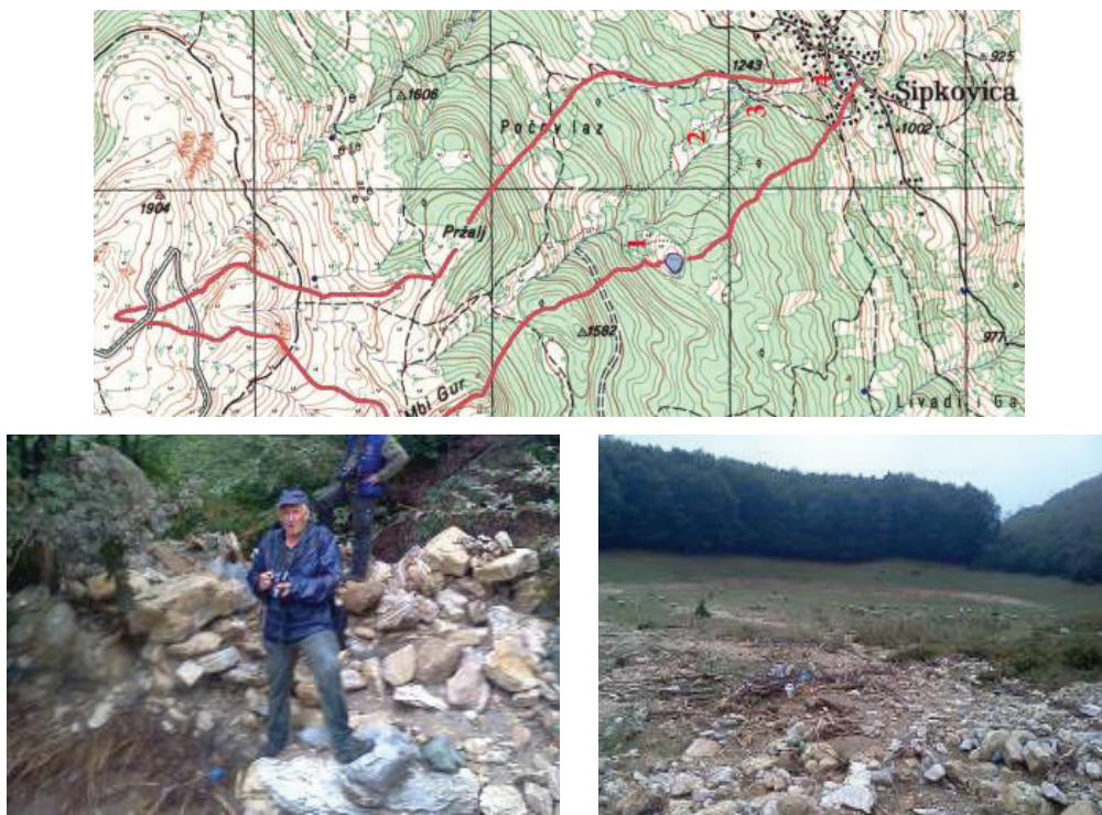
Figure 11. Šipkovicva central torrent- catchment area- Collapsed dam (1) and sinkhole (2)
